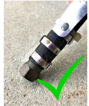
Figure 7 No Sign of Moisture or Discoloration
