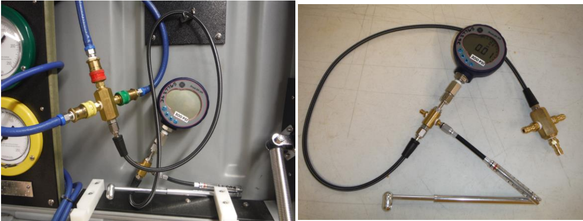
Figure 18 300 psig digital gage installed for pneumo testing
