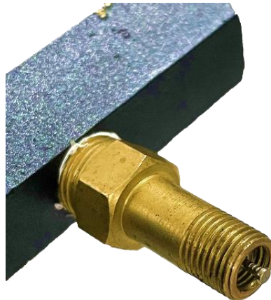
Schrader vent tip sticking out – for venting only
